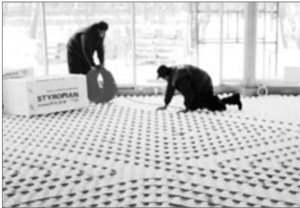
The floor heating arranged with the wet method - heating pipe direct pouring in floor pavement.
