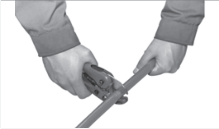
Cut PE-RT or PE-Xc pipe of required length using shears. Cut perpendicularly to pipe axis.
